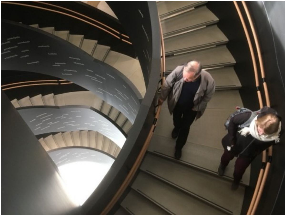
Staircase with double handrails at different heights – one for children and the other for adults
